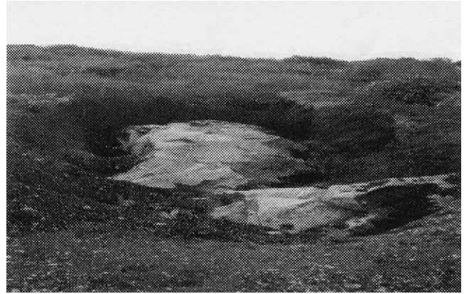
Fig. 2. Exposed rock ready for heat treatment, Chilenje South, Lusaka.
